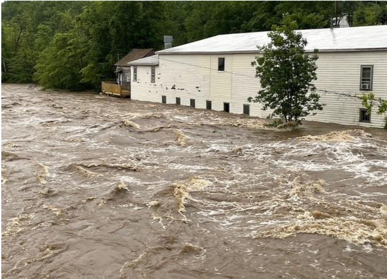
Above: Forbes Construction building on July 10, 2023; Source: Town of Londonderry.
